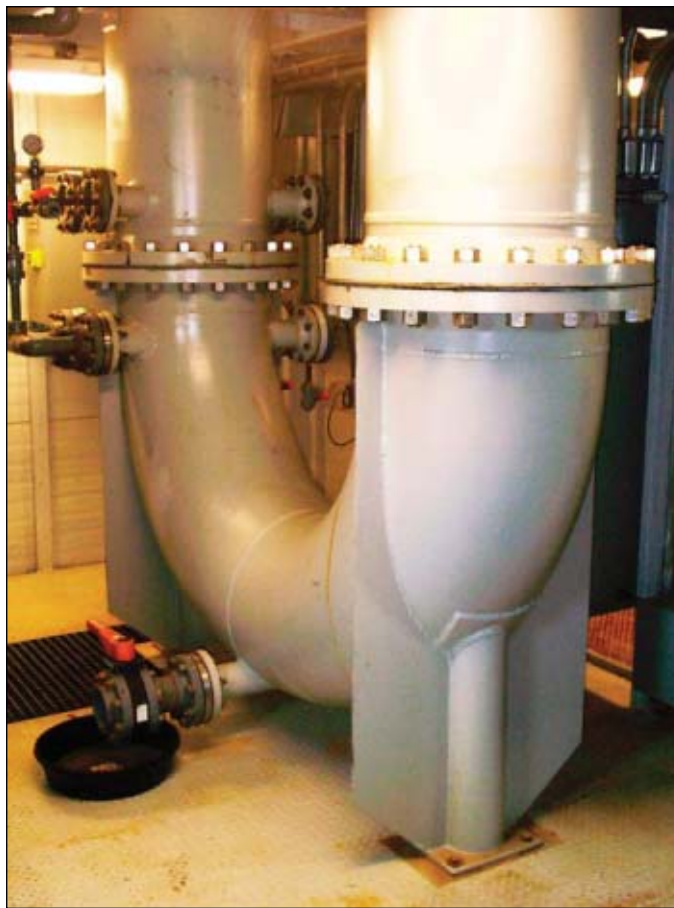
Na-loaded resin regeneration takes place in the bottom of the Higgins Loop (Fig. 2).
